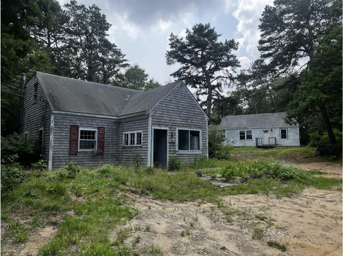
Two cottages slated for demolition. Photo by Stephen O'Grady.
